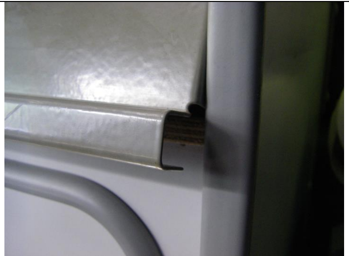
Faceplate is pulled away so that it will slide down and clear the plywood
