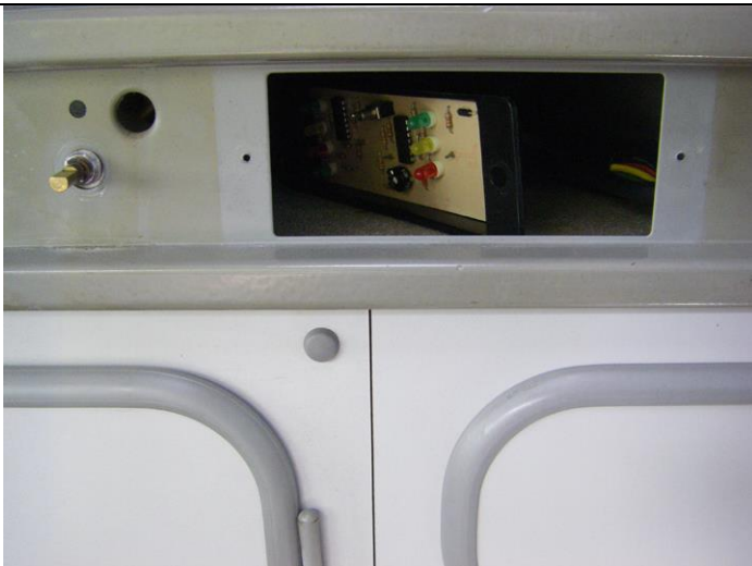
Set the LED panel inside the stove
