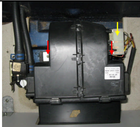
Remove the white electrical connector (yellow arrow). Remove the two blower assembly screws from the floor (red arrows). Note: There is a block of wood under each bracket that may be soaked in coolant.
